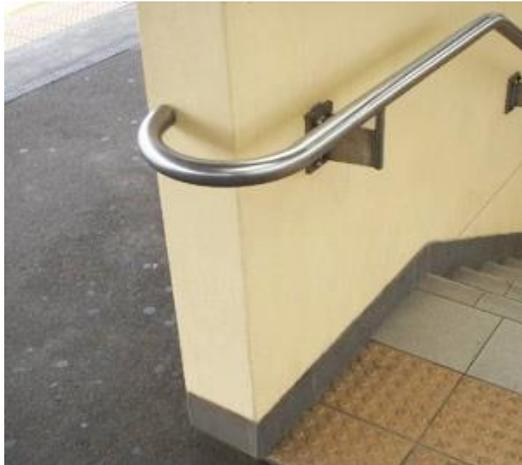
**Figure 7.5: Compliant, stair hand rail with return to the wall**
