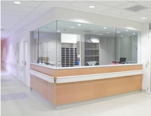
**Figure 4.5: Staff Station with security glazing barrier**
