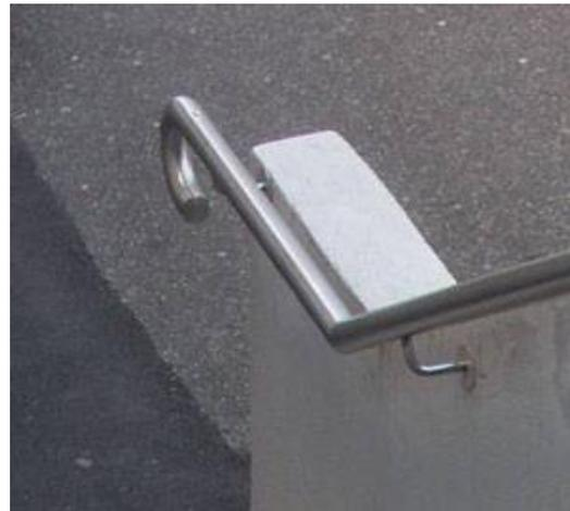
**Figure 7.6: Compliant, rail extends beyond the stair**
