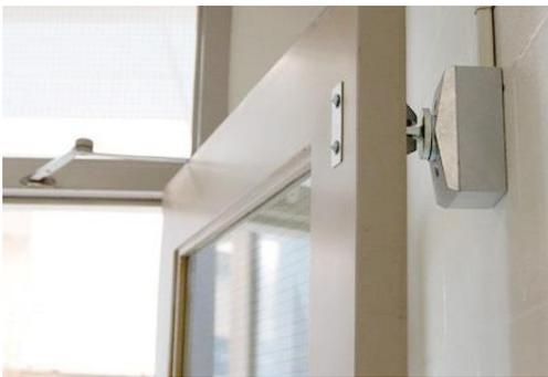
**Figure 6.9: Electronic operated door hold-open device**
